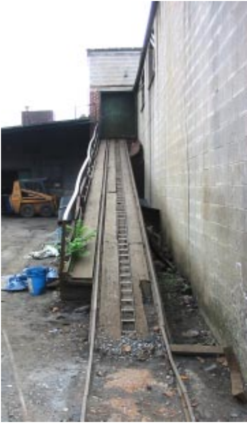
Photo 4. Views up and down the rails for cable car used to transport materials from ground level up to the cupola charging platform.
