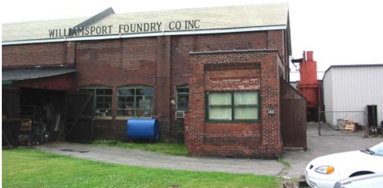
Photo 1. Office and pattern shop at the Williamsport Foundry. (Building in background is for storage.)
