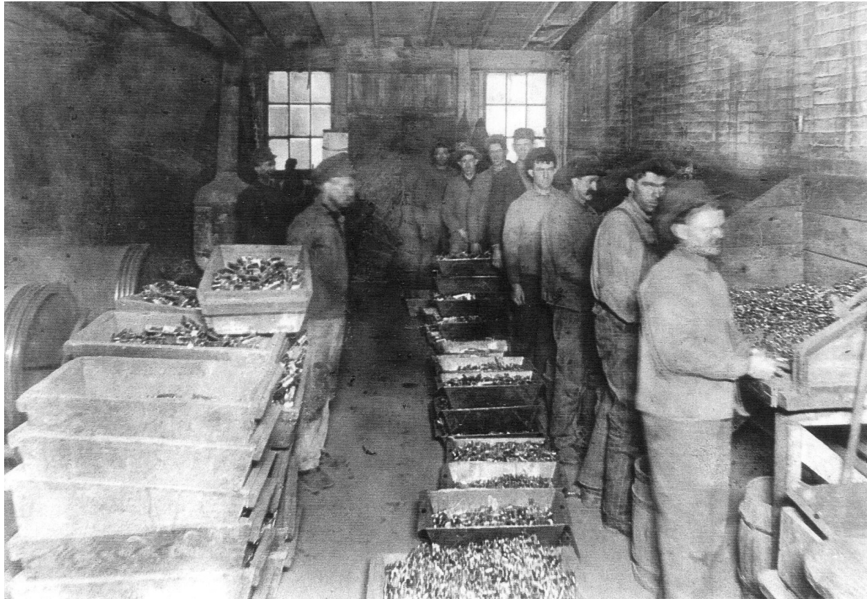
Figure 5. Tumbling Shop of the Kenton Hardware Co. in 1913. To the far left (only partially in photo) are two tumbling barrels that were loaded from the ends and rode on two rotating shafts. At far right workers are separating parts from tumbling stars. Notice how bright the parts appear. Photo provided by Robert Saylor.
